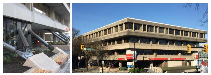
Figure 1. Two pairs of V-configuration BRBs and four inclined BRBs on each side of the building, external to the building (seven of eight on one side in left photo; BRBs visible in lowest floor, left portion in right photo).
